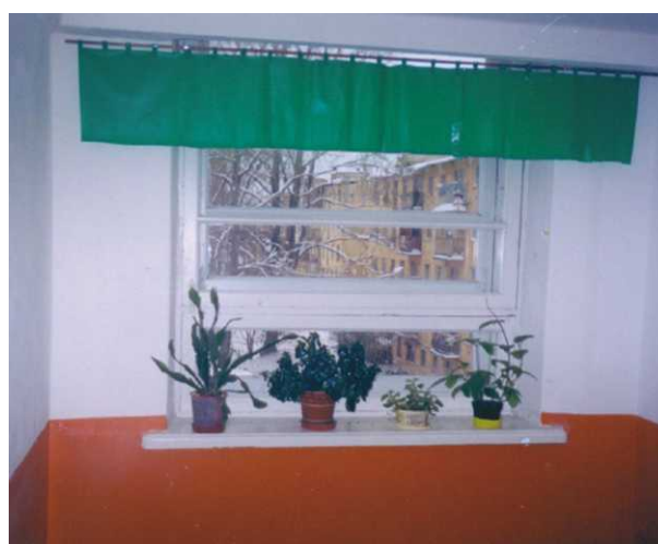
Window after repair in Petrozavodsk
