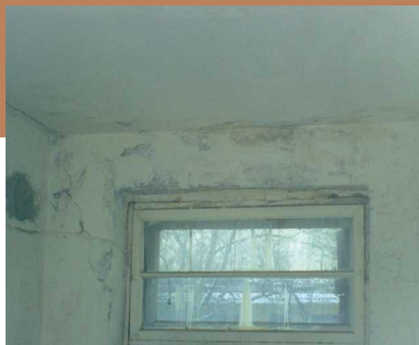
Window before repair in Petrozavodsk
